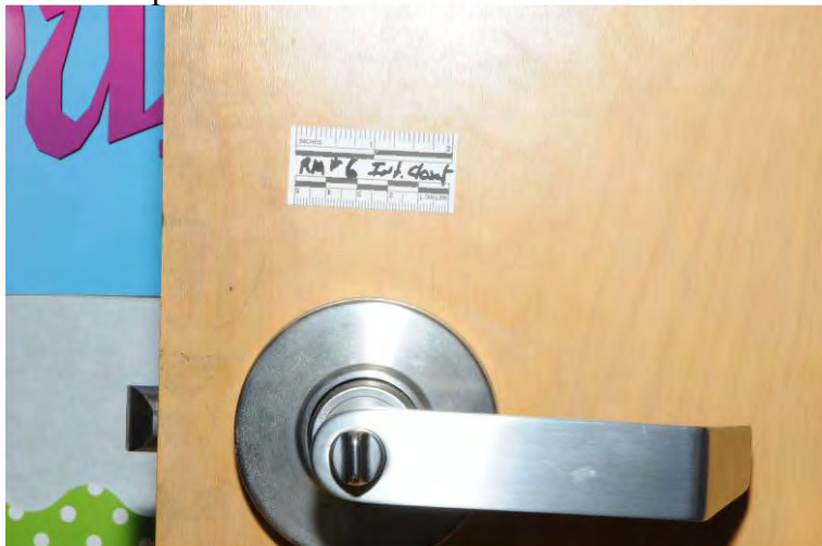
134 Example classroom closet door lock – interior
