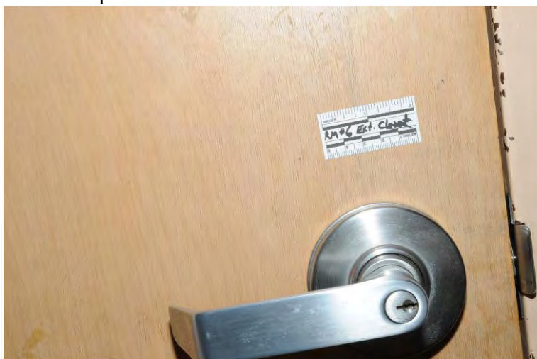
135 Example classroom closet door lock – exterior
